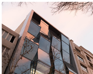
Golazin Building Location: Sari, Client: Arsh Pooya
