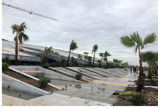
Saeed Trade Center Location: Sari, Client: Arsh Pouya, Under Construction
