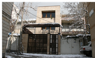
Architects Office Location: Tehran, Client: Taraghijah
