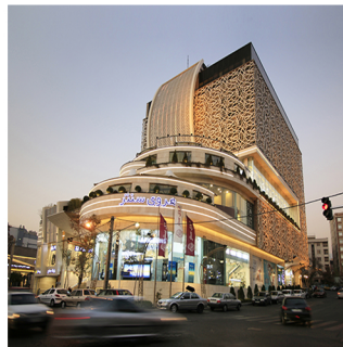
Heravi Center Location: Tehran, Client: Seyfan
