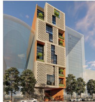
Bokharest Building Location: Tehran, Client: Tehran Chemie Pharmaceutical Co., Under Construction
