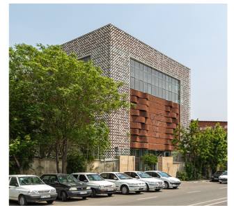
Henkel Building Location: Tehran, Client: Tehran Chemie Pharmaceutical Co..
